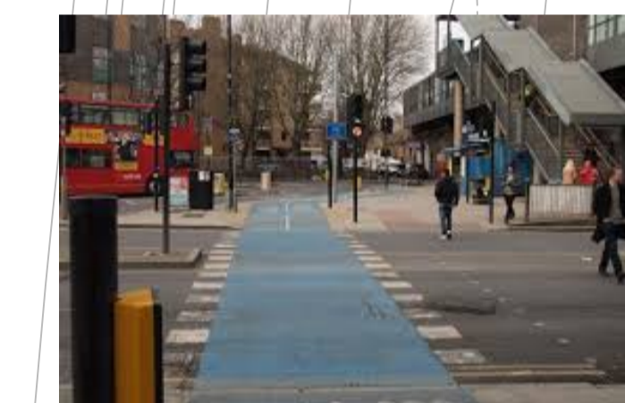
A simple (and economic) signalled parallel crossing in London
