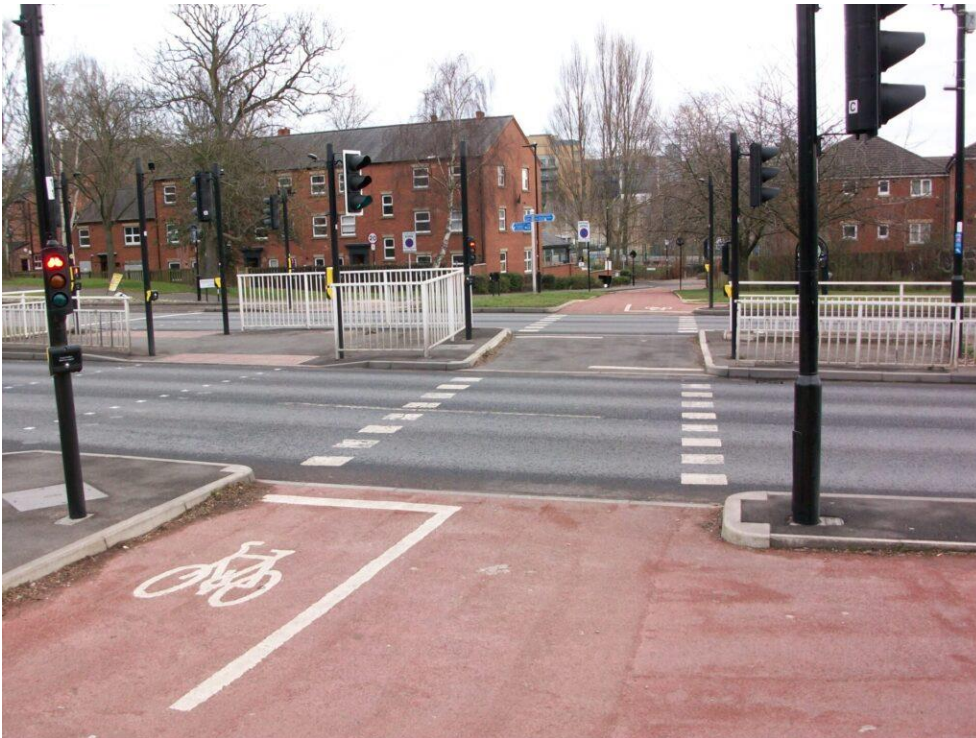
Figure 2: An example parallel signalised crossing in Sheffield.
